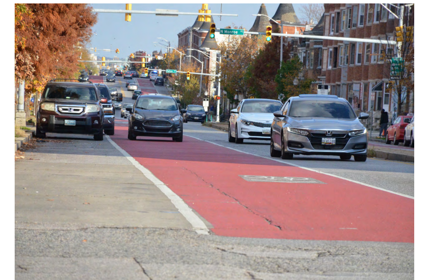
Figure 23 Cars driving along West North Avenue, including in the red-painted dedicated bus lane.
