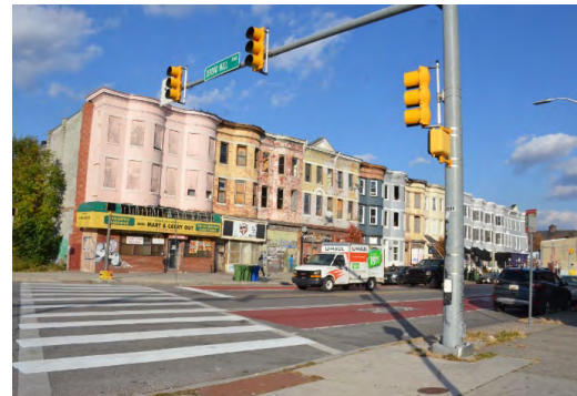
Figure 40 Commercial first floor
